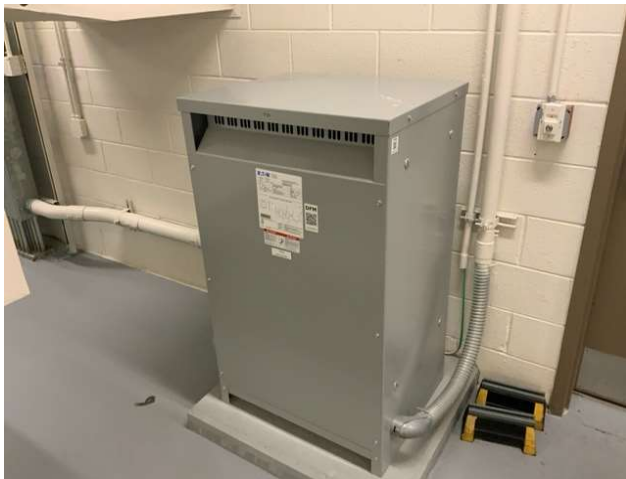
27 - SECONDARY TRANSFORMER
