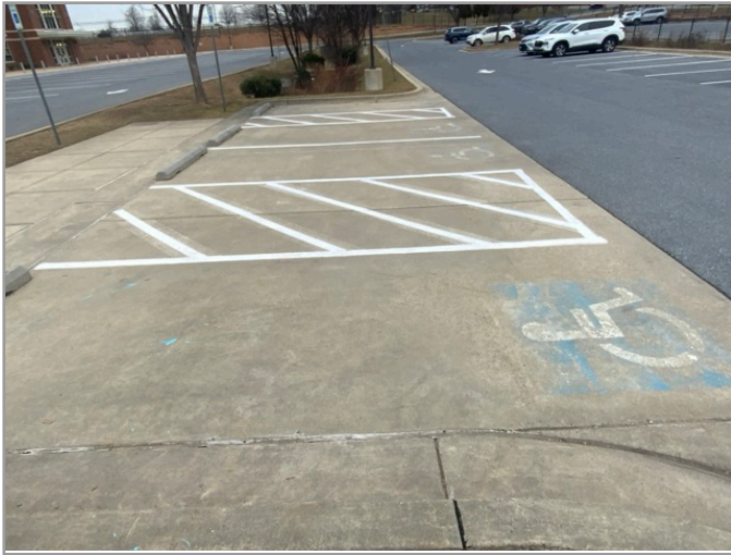
OVERVIEW OF ACCESSIBLE PARKING AREA
