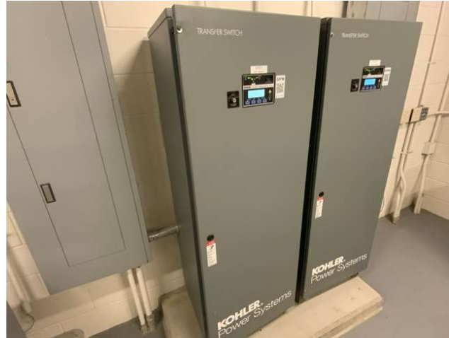
26 - AUTOMATIC TRANSFER SWITCHES
