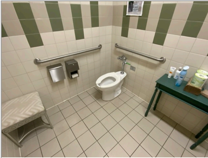
TOILET STALL OVERVIEW
