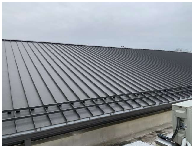
6 - STANDING SEAM METAL ROOFING
